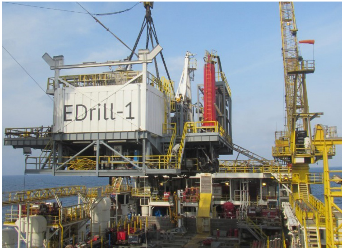
Lifting of a drilling module onto the host platform.
