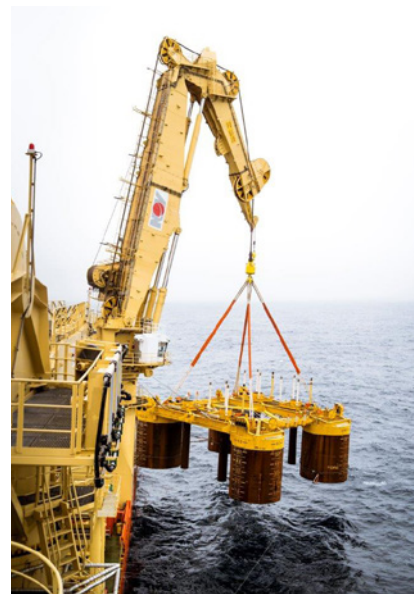
Installing a subsea template
