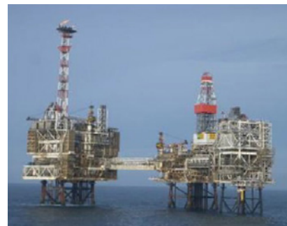
The Etap platforms
