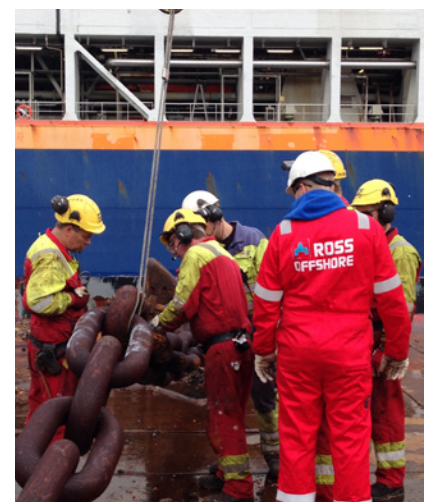
Ross Offshore planning and supervising mooring chain replacement at the Åsgard A FPSO.
